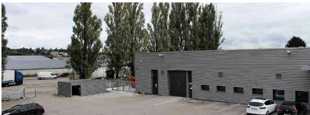
Figure 2. Le datacenter Tier III+ EcoBreeze Franc-Comtois.
